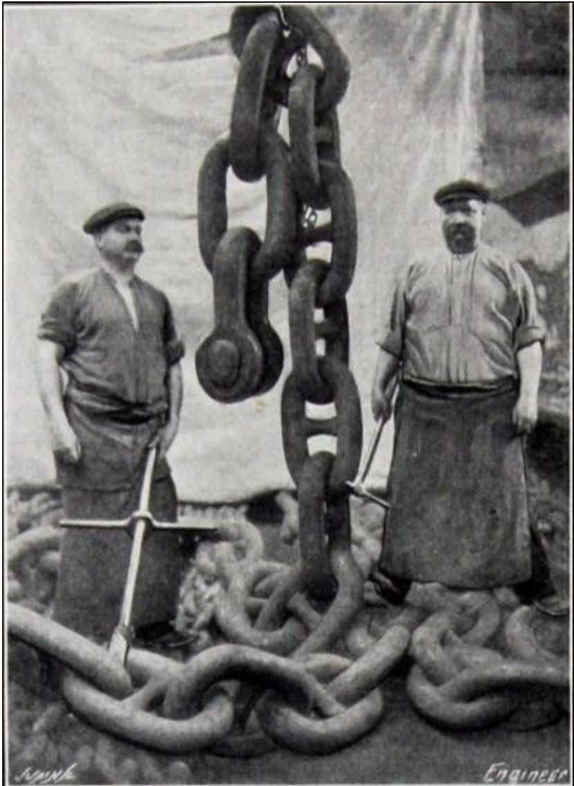
Another great cable made at the Newbridge Chainworks of Brown and Lenox in 1906.
